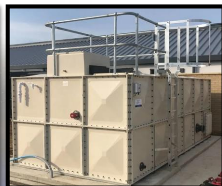
Actual Sample photo of Fire Sprinkler Tank
