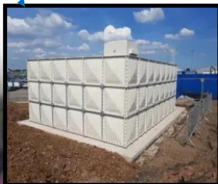
Actual Sample photo of Fire Sprinkler Tank
